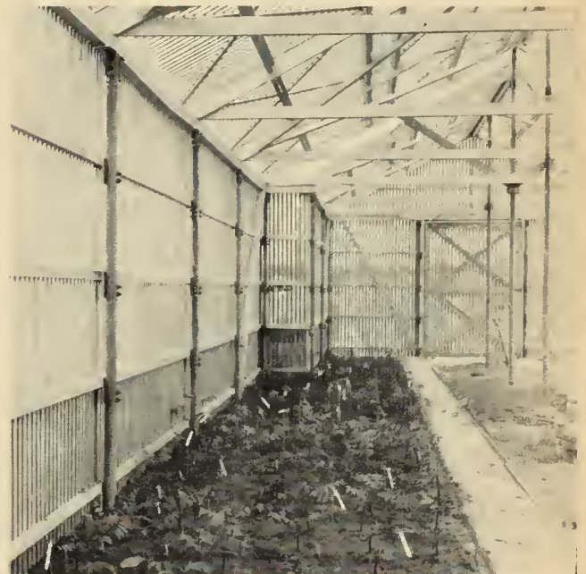
Detail of lath house.
